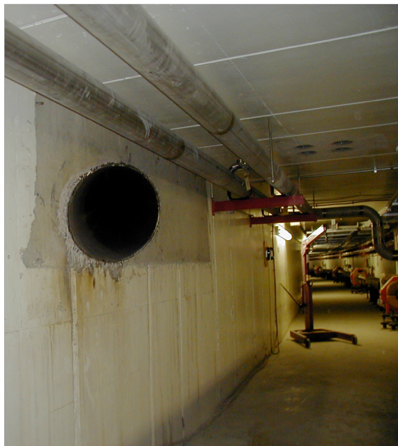
Figure 2: End of carrier pipe where it penetrates the wall of the Main Injector tunnel. This pipe was installed to enclose a low-energy beamline from the Main Injector at MI-10 to the experimental hall at MI-9. The four penetrations on the ceiling also lead to the location of the future MI-9 enclosure.
